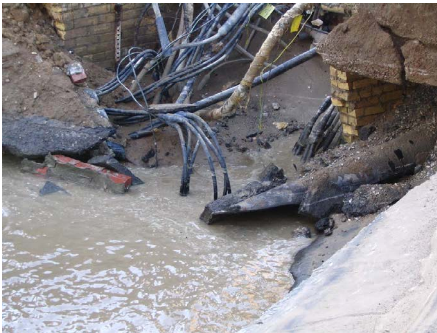
Figure D-4: Spiral watermain break with evident Contamination .
