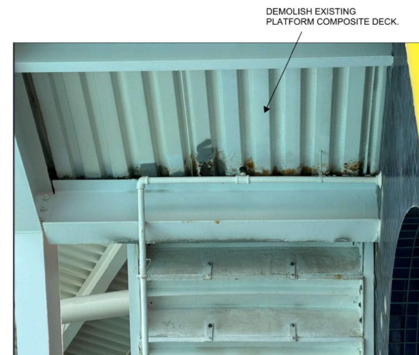
FIGURE 1: VIEW SHOWING THE EXISTING PLATFORM SCALE: N.T.S
