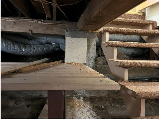
Figure 19: Wooden beams supported by concrete column.
