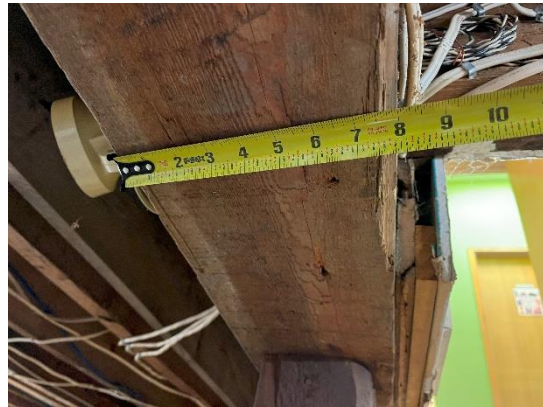
Figure 22: Wooden beams measured to be 8"x6".
