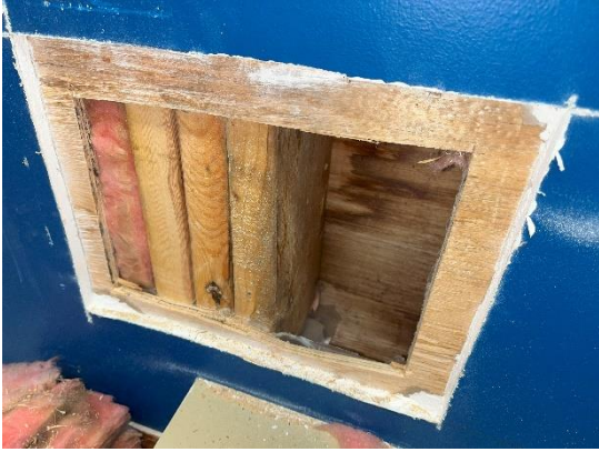
Figure 05: Additional stud framing provided under windowsill.
