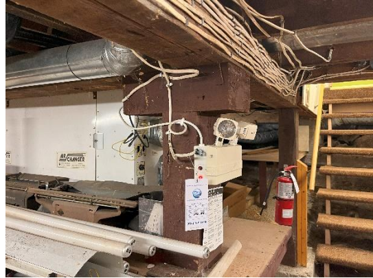
Figure 20: Wooden beam supported by wood posts.
