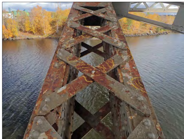
TYPICAL PHOTO OF LATTICE BARS
