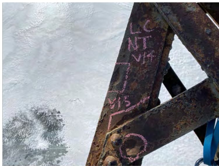
TYPICAL PHOTO OF SEVERE SECTION LOSS IN TOP FLANGE OF LOWER CHORD.
