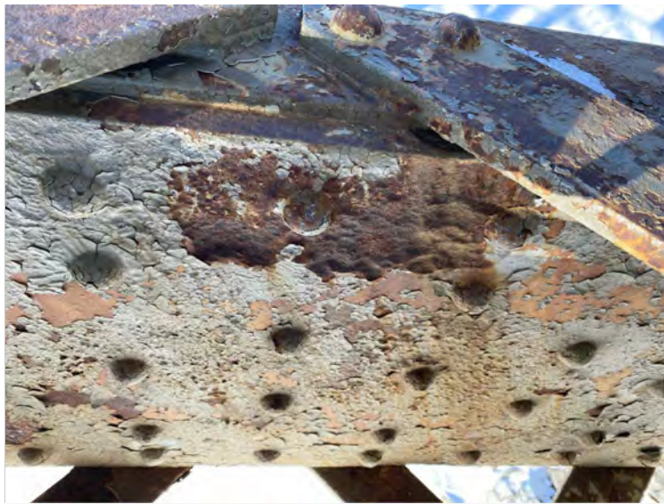
TYPICAL PHOTO OF SEVERE SECTION LOSS IN WEB OF LOWER CHORD.
