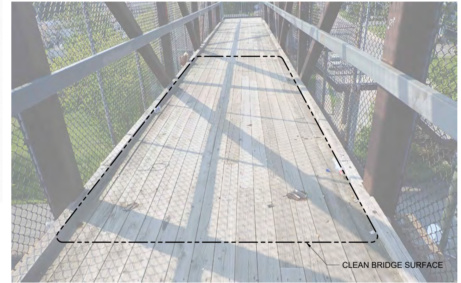
1 DECK MAINTENANCE DETAIL NTS
