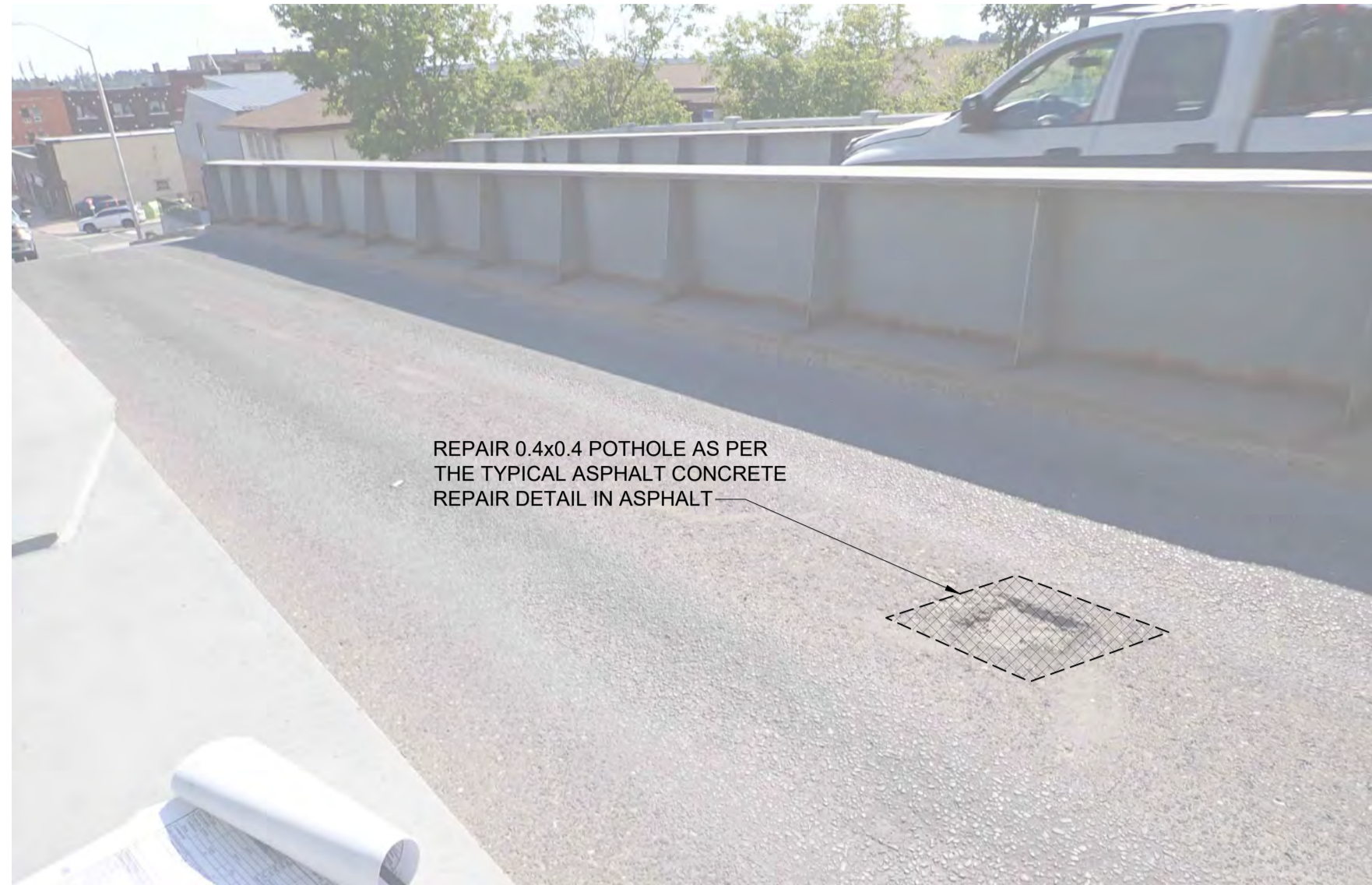
1 NORTHBOUND LANE - DECK DAMAGE DETAIL 11 12 NTS
