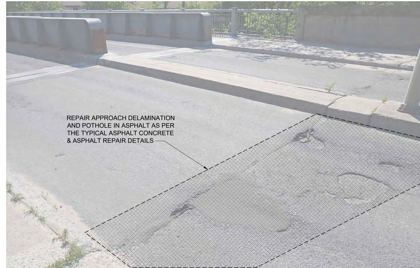
2 NORTHBOUND LANE - APPROACH DAMAGE DETAIL 11 12 NTS
