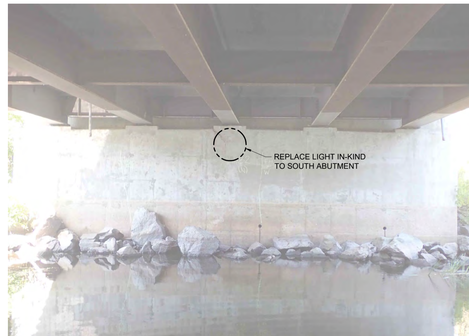
ELEVATION - NORTH ABUTMENT NTS
