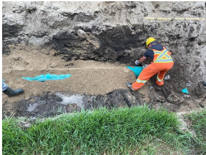
Storm Repair Ottawa St Keewatin
