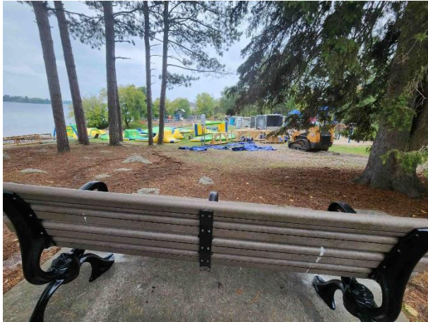
Donation Bench Installation
