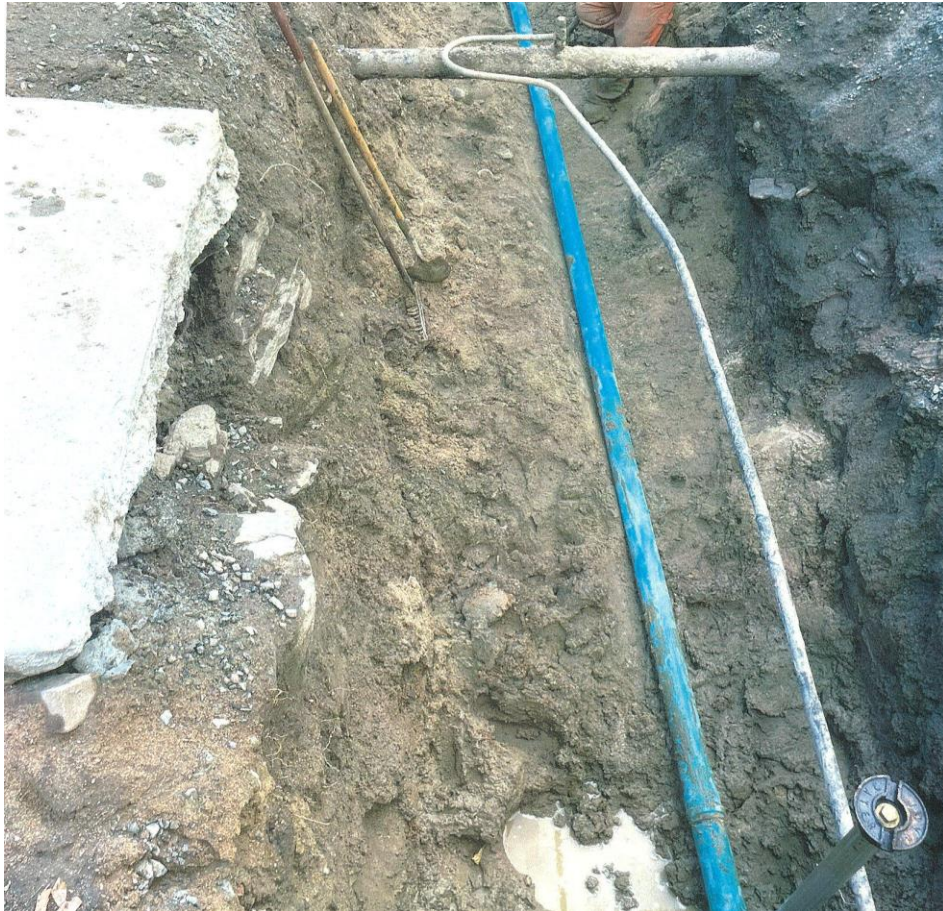
7 th Ave S Wastewater Break Repair
