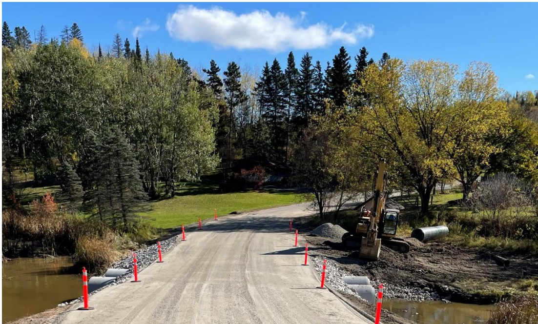
Gould Rd Culvert Replacement
