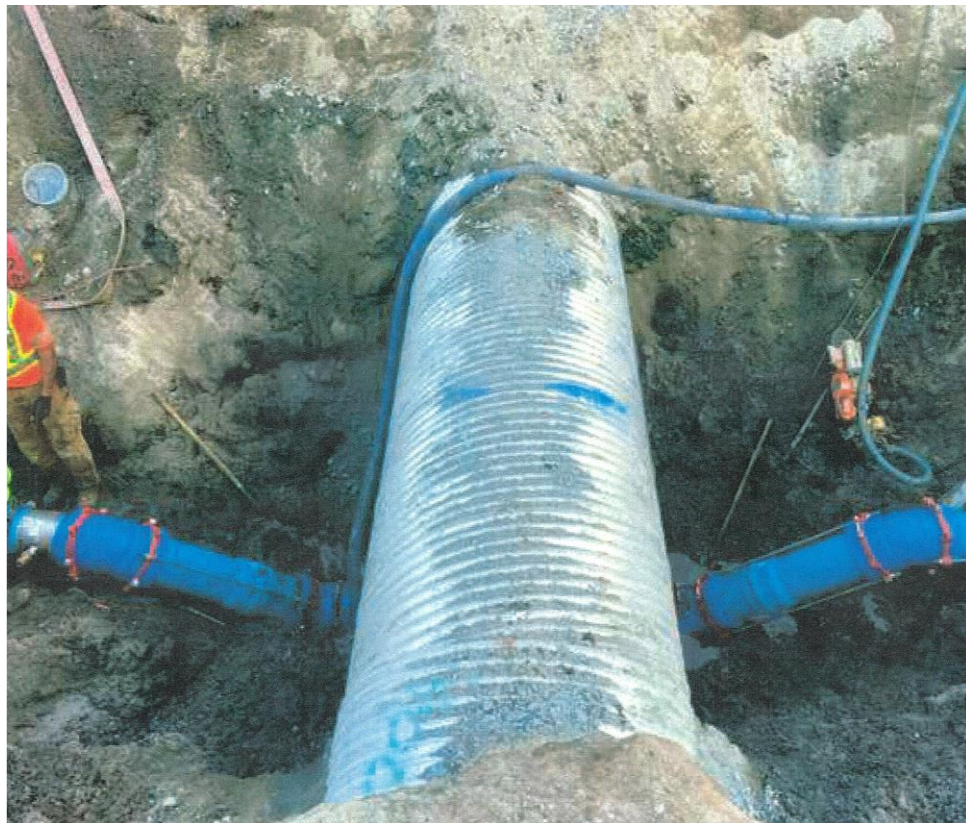
9 th St N Main Break Repair
