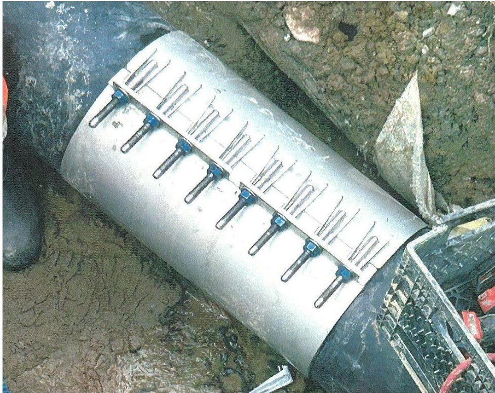
1 st Ave S Main Break Repair
