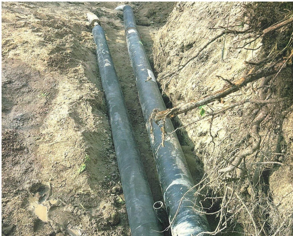
6 th Ave S Wastewater Break Repair
