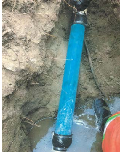
Beach Road sewer service repair
