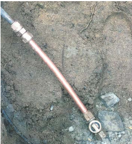
Beach road service repair
