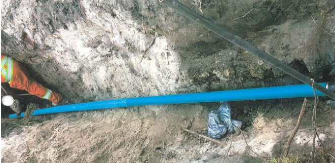
Matheson Street North sewer service repair
