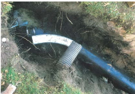
5 th Street North sewer main replacement
