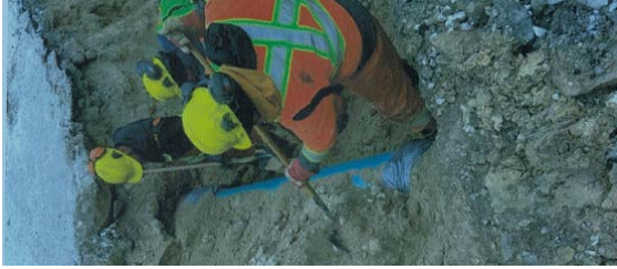
Regina Ave sewer repair
