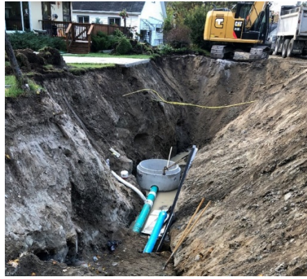
Figure 1: Construction proceeding on 7th Avenue South
