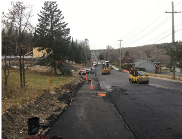
Figure 2: Ninth Street North paving
