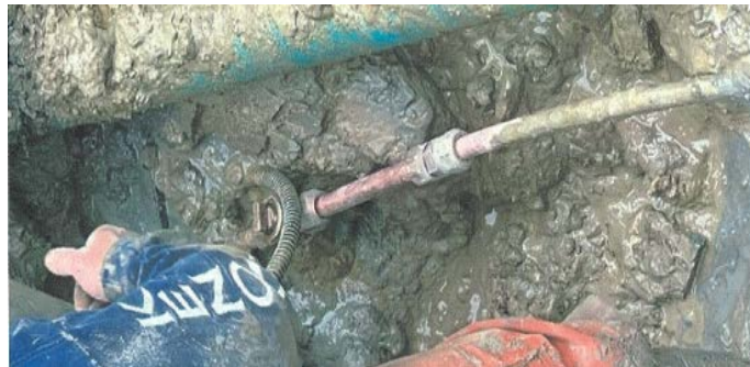
Donbrock Drive service box replacement
