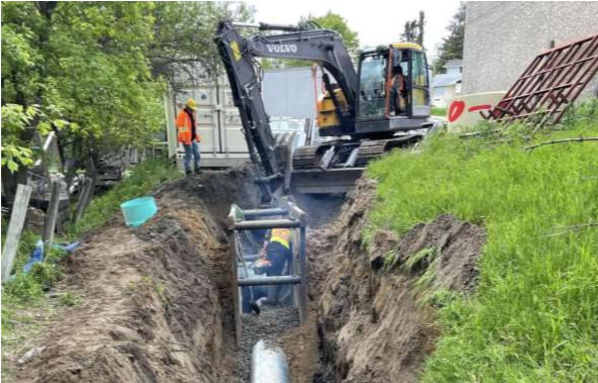
*Figure 3: The excavation required the use of a trench box to protect workers.*
