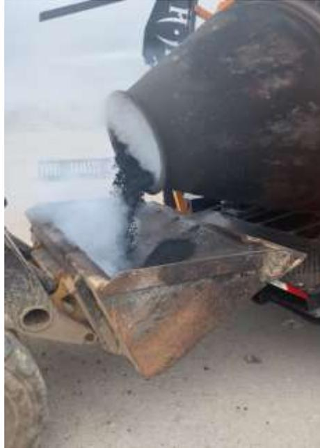
Dumping of the transformed Asphalt chunks into hot asphalt
