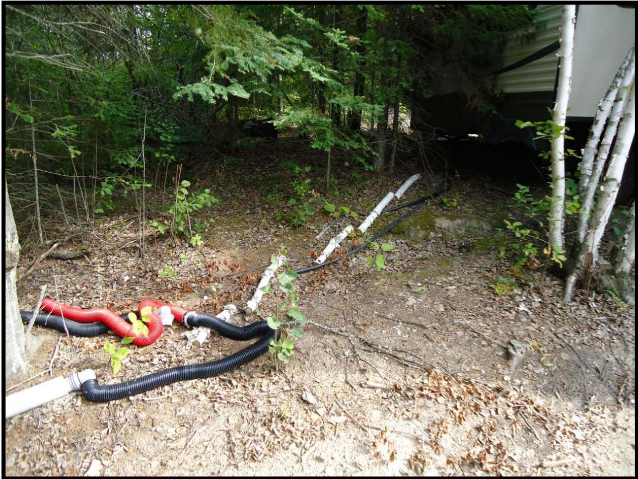
**Figure 4:** Wastewater lines connected to campers on the property
