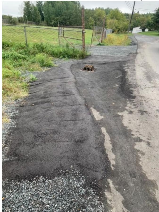
Manhole repairs Shauna Crescent, asphalt still required.
