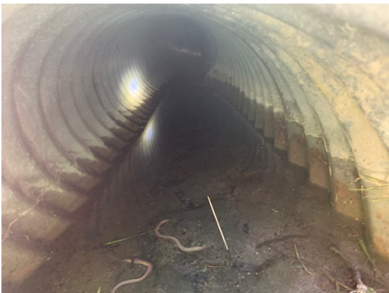
Before Culvert Flush
