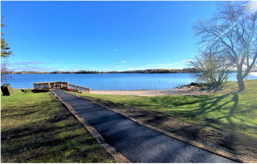
Coney Island Footbridge island side abutment upgrade
