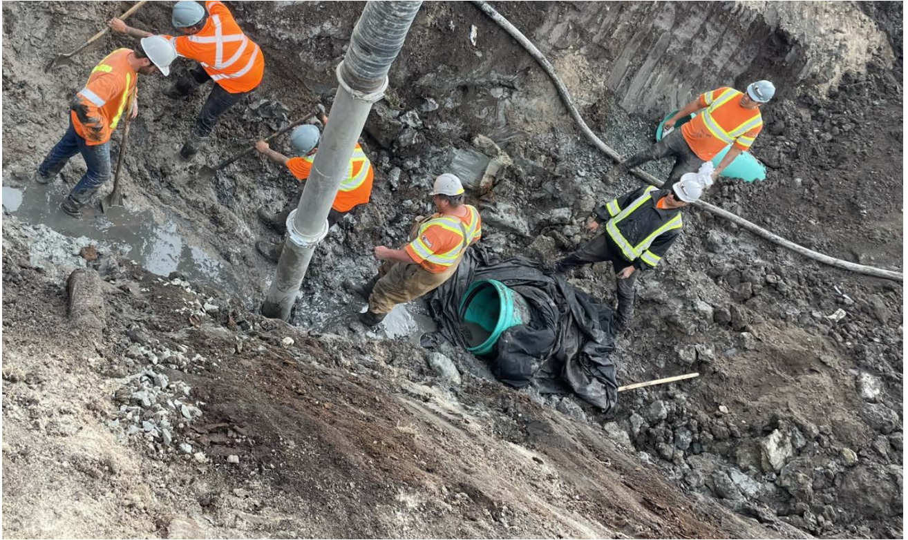
Figure 1: Central Park - Geotextile Installation and Ground Water Infiltration
