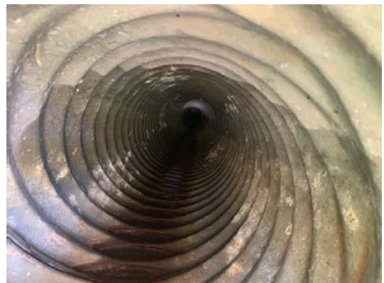
After Culvert Flush
