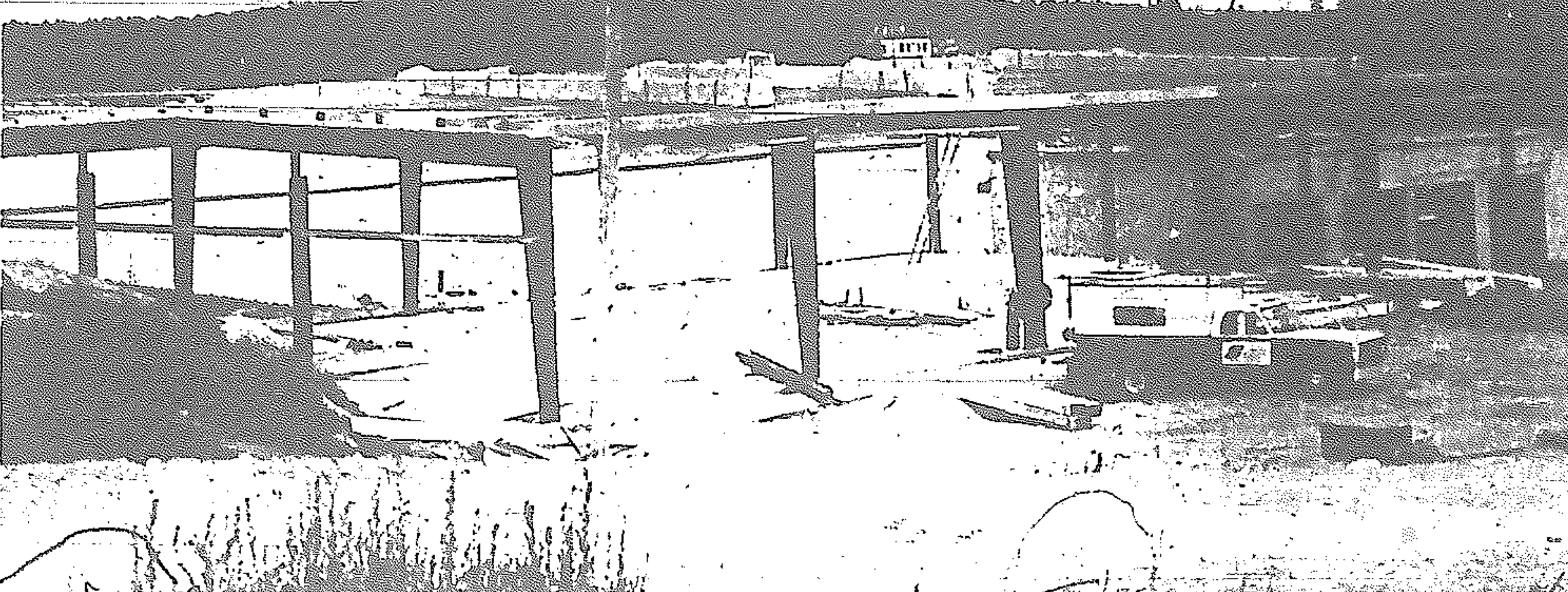
GARAGE CONSTRUCTION —Work is progressing on the construction of a new garage for the town of Keewatin. General contractor is Sillman Construction Company of Thunder Bay. The $40,000 garage is scheduled for completion within the next month and is located on municipal property, overlooking Darlington Bay. (Staff photo)
