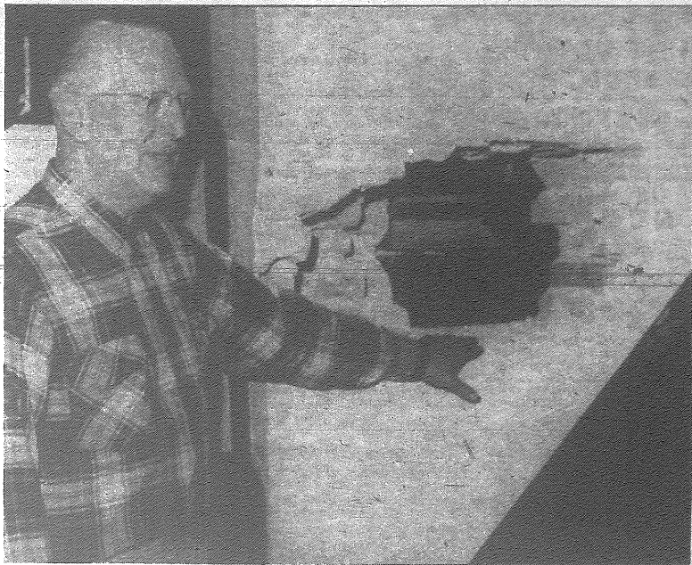
ERNIE NEWMAN POINTS TO HOLE SMASHED IN BRICK WALL BY BURGLARS WHO ATTEMPTED TO GAIN ENTRY TO THE STORE VAULT.
