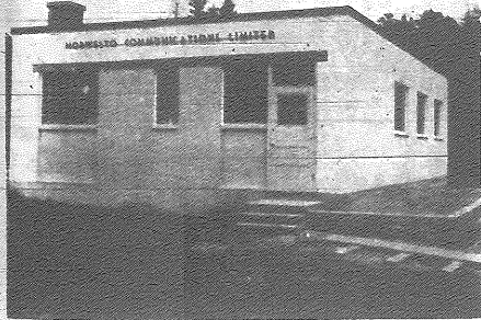
This well-constructed building houses the new dial automatic exchange which Norwesto puts into use June 7th for Jaffray-Melick subscribers. It is located near the east end of Rabbit Lake.
