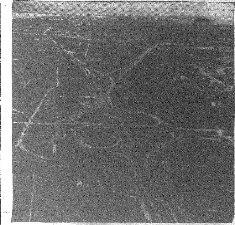
Modern highways must provide a smooth blending of communications between city and country. The Freeman by-pass and interchange on the Queen Elizabeth Way near Hamilton is an integral link in such a system.
